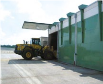
Dry digestion biogas plant
